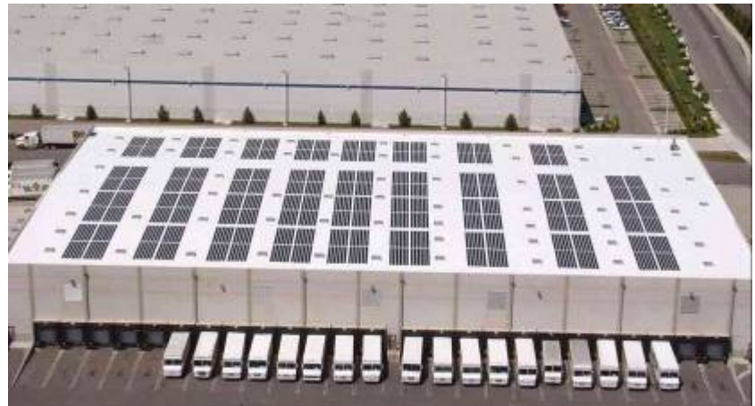
100 kW EV Charging and H 2 Production
