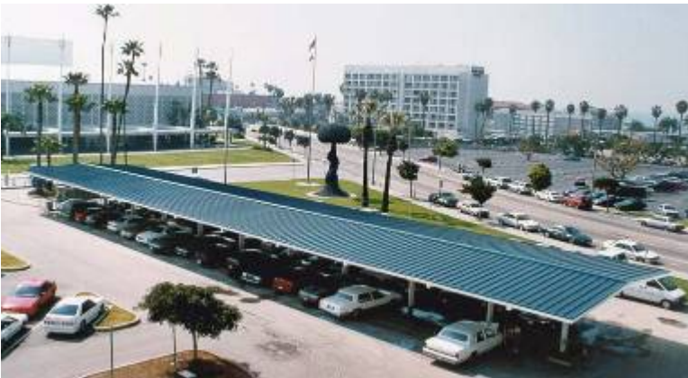
30 kW EV Charging Shade Structure
